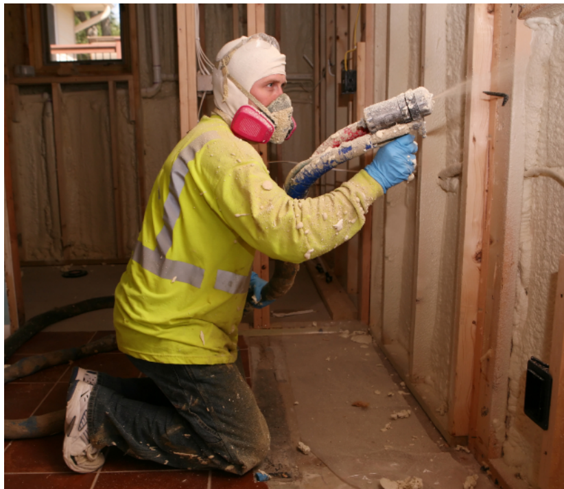
A contractor sprays insulation during a retrofit job
