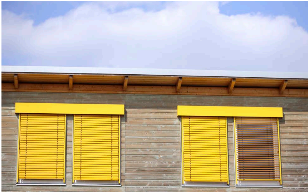
Window treatments can help keep a building cool even during hot weather
